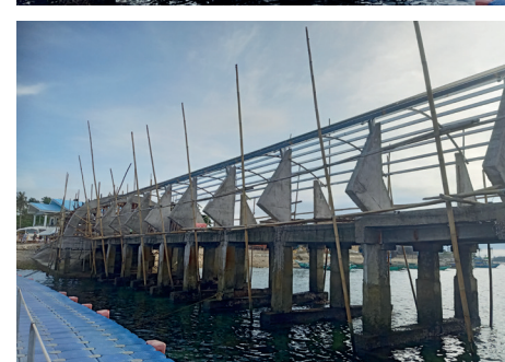
Tabon jetty port under construction (Photos by Adrian Magsipoc)
