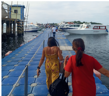
Tabon jetty port pontoon bridge traveling from Caticlan to Boracay
